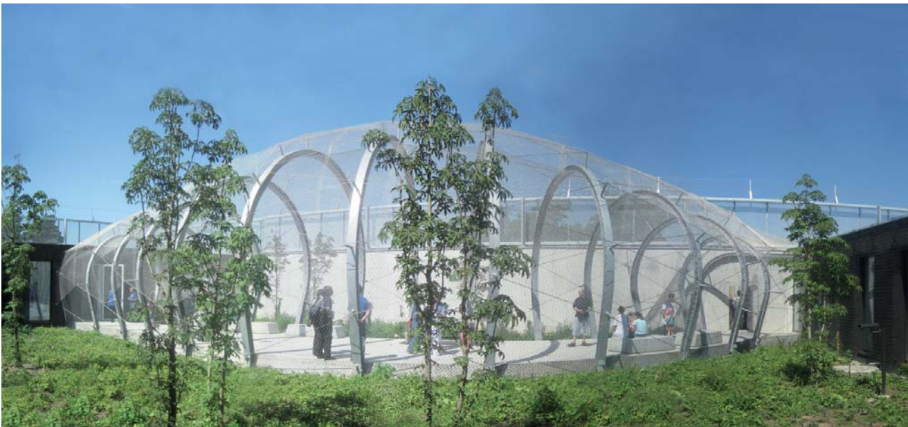
One of the three walkways surrounded by ROMBO high-tensile steel wire mesh
